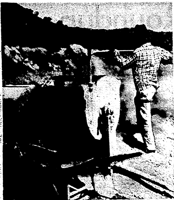
ADOBE BLOCK is made much the same as it was in days of old, although there have been refinements, mainly the addition of an oil emulsion to make adobe waterproof and resistant to deterioration. The formula is mixing the soil with water and emulsion, (above) then pouring it into forms to mold the block, (below) and then letting it cure in the sun, turning the block on edge after it hardens (bottom). This is the handcraft method. Most modern adobe plants now produce the block in uniform size and shape by machines.
