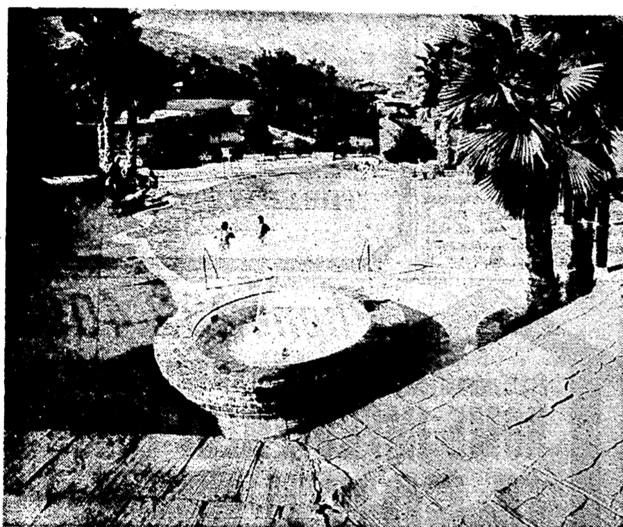
ADOBE BUILDINGS and walls enclose central recreation area at all-adobe Pala Mesa Village. Circular fountain, however, is fashioned from ornamental used brick for color accent. Roof, foreground, is adobe tile made at the site.
