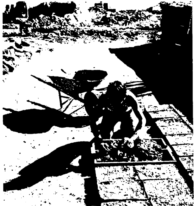
Figure 11: Tamping adobe mud into corners of wooden form at Eloy Montano's adobe yard in Santa Fe, N.M.
