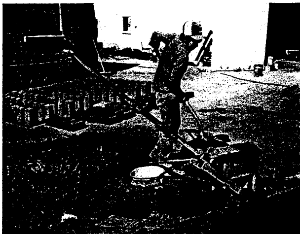
Figure 15: Use of a CINVA-Ram in the production of pressed-earth-blocks at Columbus, N.M.
