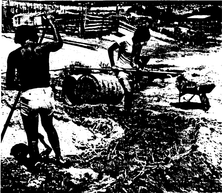
Figure 7: Mixing the mud, straw and water for traditional adobes at Nambe, N.M.
