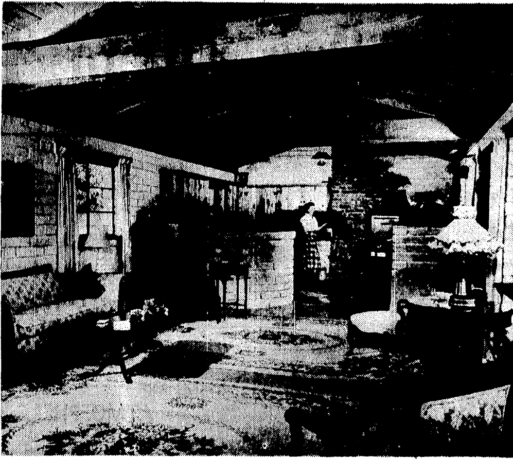
OPEN PLANNING: Even the partial partitions dividing living room from the kitchen are adobe in the Escondido home of Mr. and Mrs. B. William Sinclair Jr.
