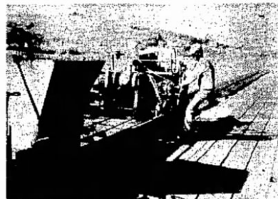
"Mother hen" machine lays 20 adobe blocks at a setting. Blocks then "cure" in the sunshine.
