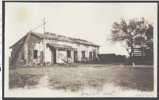
Prior to renovation
