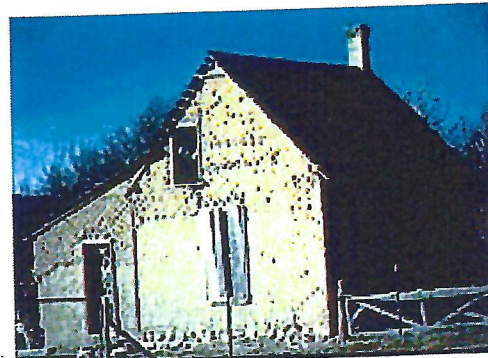
A traditional mixture of mud and straw plaster should be applied to stabilize the exterior of this house. Photo: NPS files.
