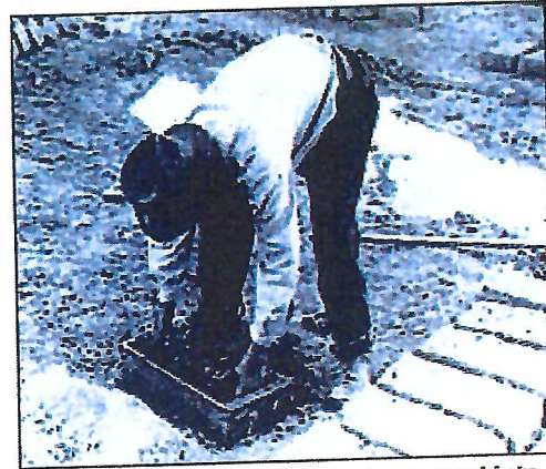
A mixture of mud and straw is pressed into a mold to form an adobe brick. After the adobe brick is removed from the mold, it must dry in the open air for a month or more before it can be used. Photo: Russell Lee, Farm Security Administration Collection, Library of Congress.
